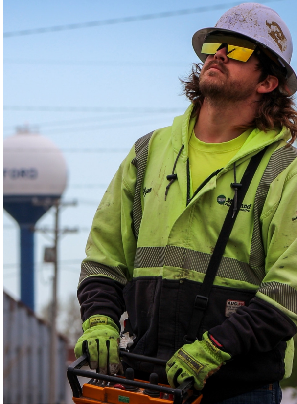
Lineman Wyatt Tharp sets a pole at Athens Woods in Stratford.
