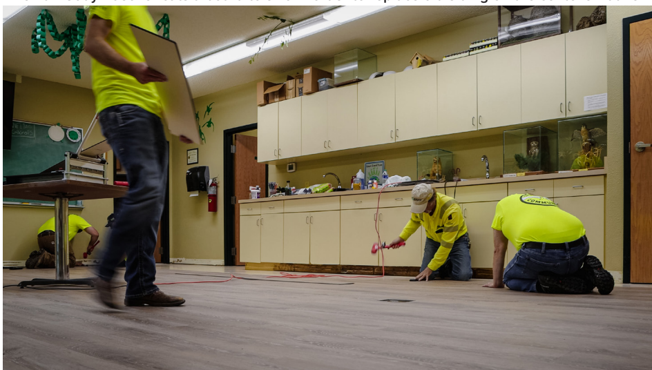
Midland volunteers helped install a new floor in the center's classroom.
