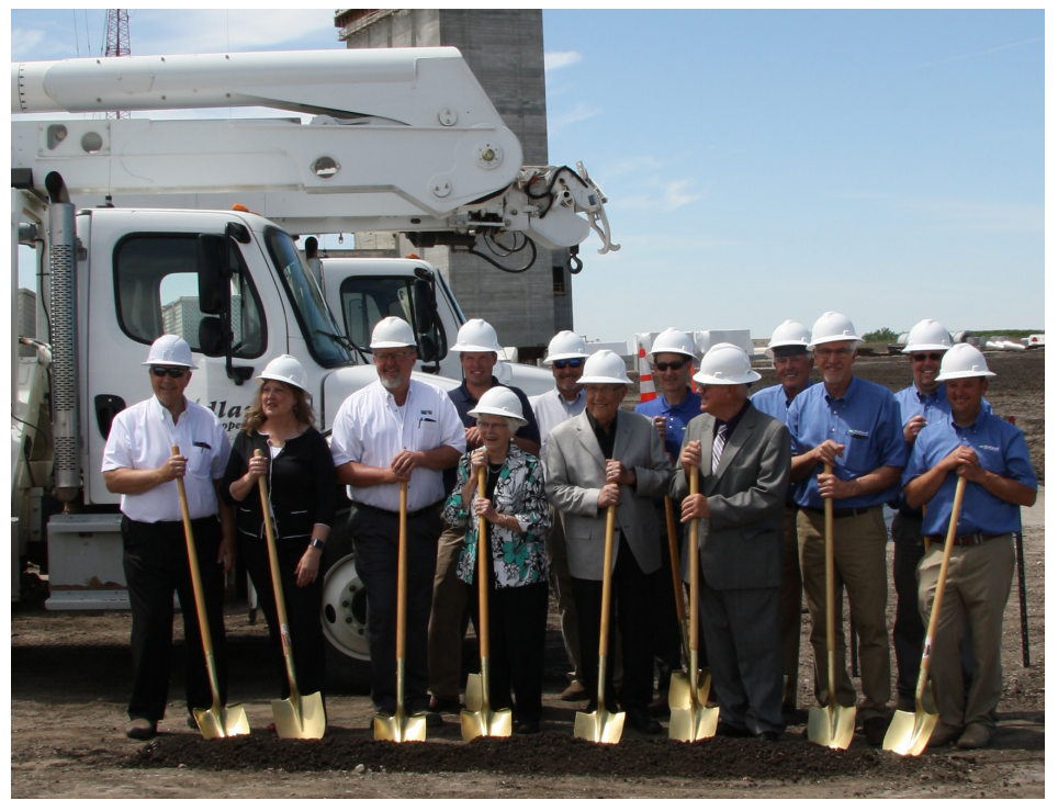
Representatives from NEW Cooperative joined Midland Power Directors and Ken Hastings' wife Pat (center left) to celebrate Ken Hastings' (center right) cooperative legacy, with a substation groundbreaking ceremony at NEW Cooperative, Cooper.
