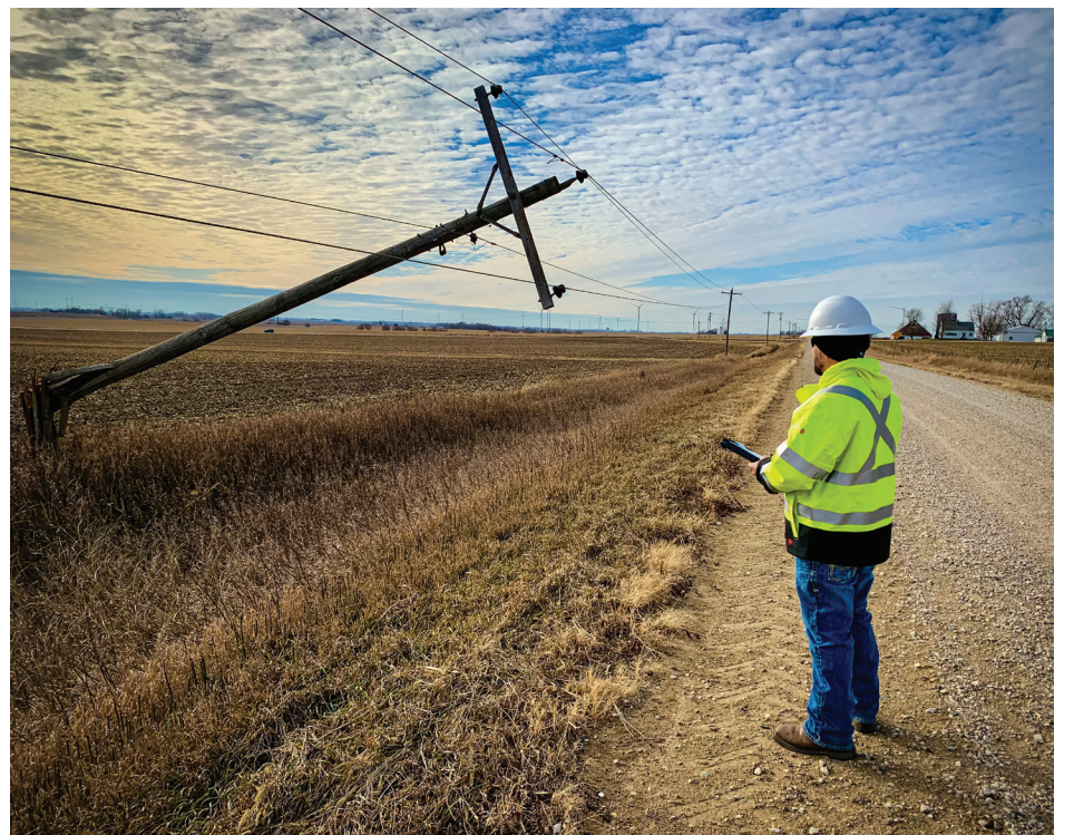
Crews initially worked around the clock repairing December storm damage.
